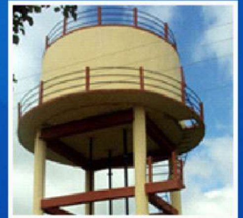
Overhead Water Tank
