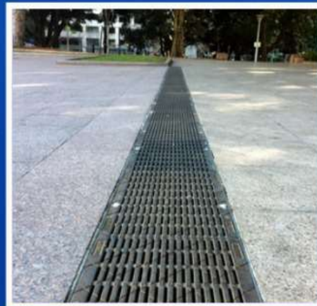
Storm Water Drain
