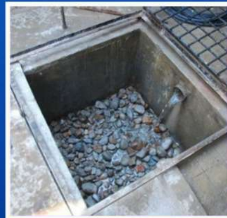
Water Harvesting Pit
